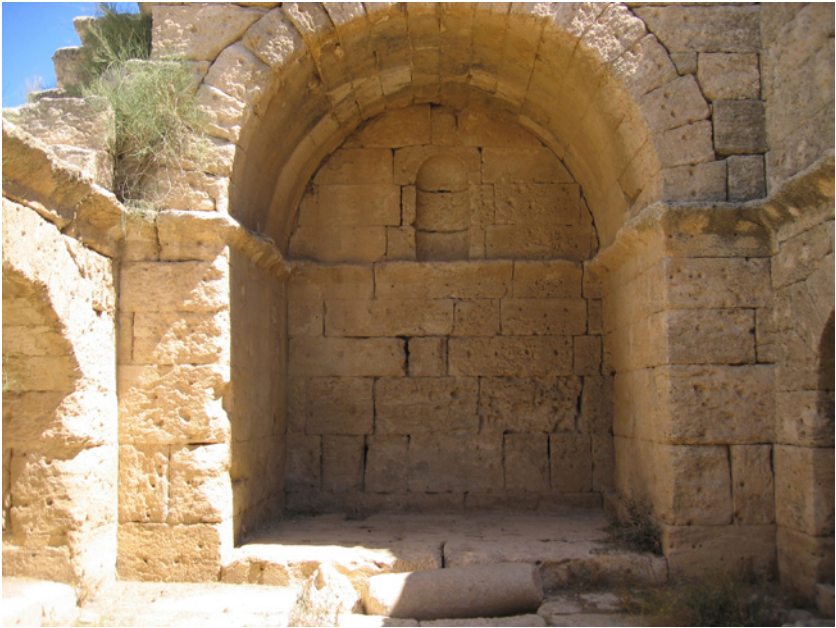
Fig. 66. Rear wall of the small temple at Dhat Ras.
