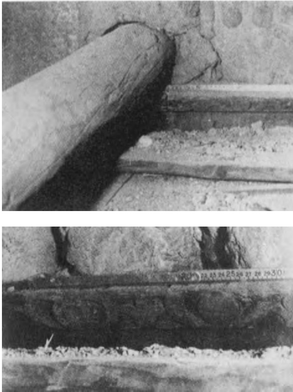
Figure 2.19 (a) View and (b) detail of a carved and painted wooden cornice (now obscured by the ceiling of the outer ambulatory), early ninth century. After Christel Kessler, 'Above the Ceiling of the Outer Ambulatory' (1964). Courtesy of the Royal Asiatic Society.
