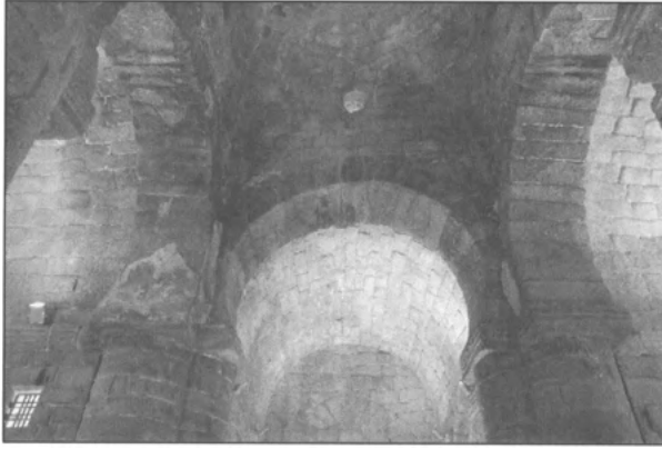
Fig. 8.9: Stone pendentive dome and vaults of Santa María de Melque (Toledo), with remains of stuccos
