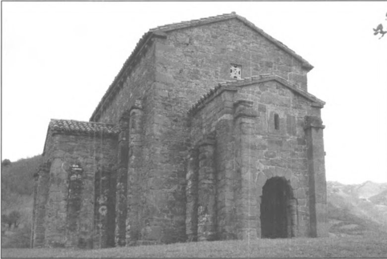
Fig. 8.8: Santa Cristina de Lena (Asturias) with ashlar stone masonry in quoins and buttresses
