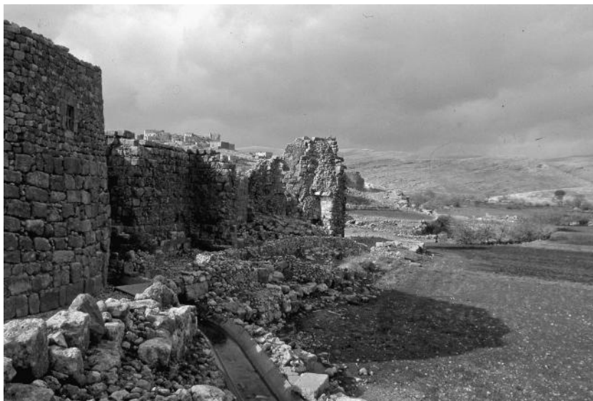
FIGURE 2.5 The walls of Dara in southeast Turkey (as seen in 1978). © Jim Crow.
