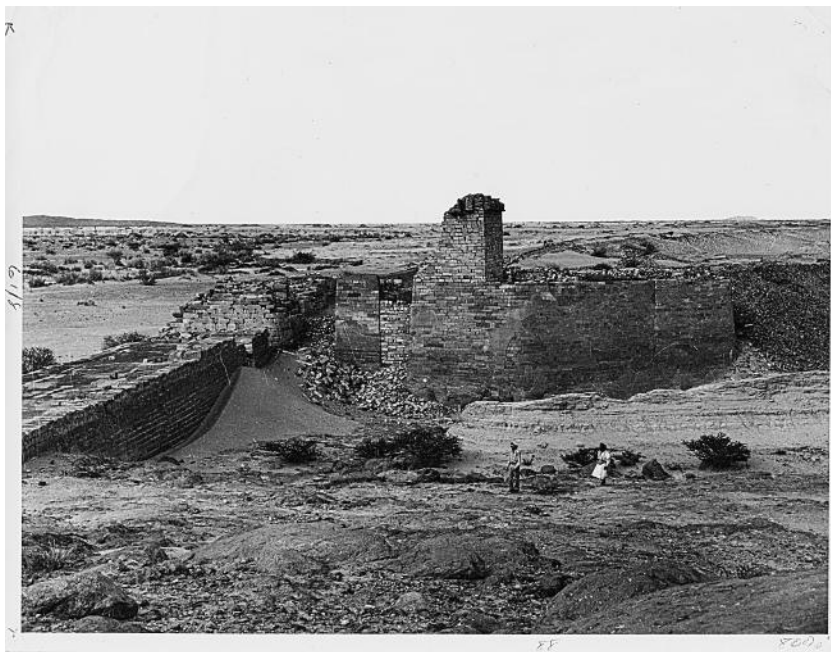
FIGURE 2.2 Dam of Marib, capital of Saba/Sheba in Yemen, northern sluice system. © American Foundation for the Study of Man.
